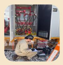
Simon performing an insulation test on the bus that feeds power to the community in Attawapiskat
