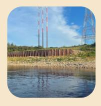
The Albany River erosion site was inspected in August for movement that may have occurred. The site was stable but the retaining wall sustained some damage from spring breakup
