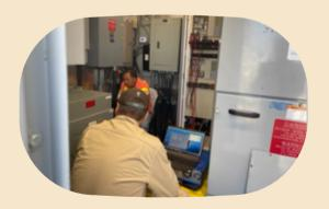
Bobby and Steven Xue, a FNEI contractor, performing a function test for a line protection relay for K5A, the line from Kashechewan to Attawapiskat
